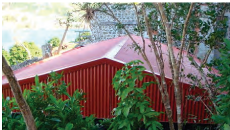
New Roof on Iron Cistern
