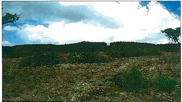
Fort Shipley Curtain Wall ~ after clearing
