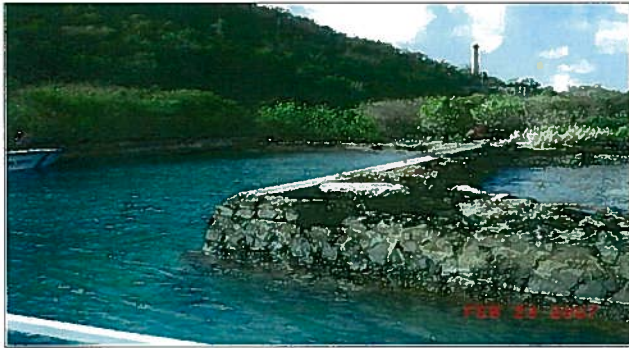
Creque Marine Railway and Head House ~ before clearing
